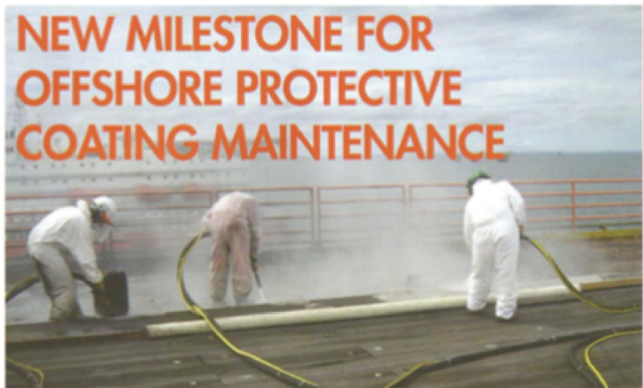
Several workers using the relatively low risk Vapour Abrasive Blasting Equipment on an offshore platform
